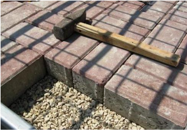
Figure (D.7): Interlock tiles sitting on top of bedding layer
