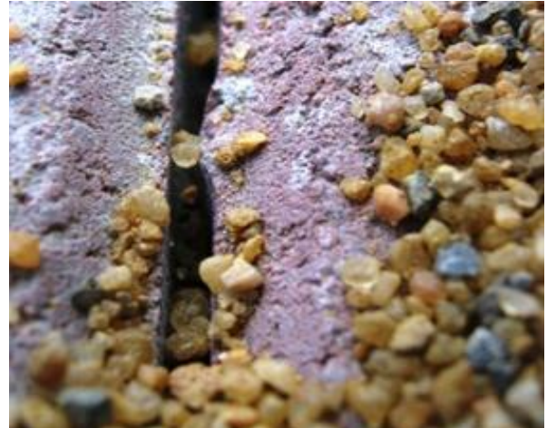
Figure (D.13): Joints between interlock tiles
