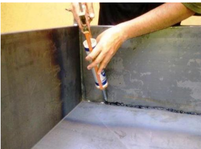
Figure (D.3): Good closing to prevent leakage of the water
