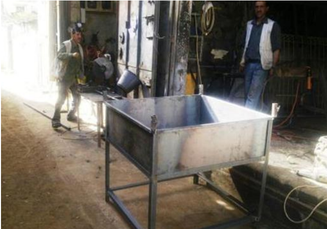
Figure (D.1): Construction of experimental steel box
