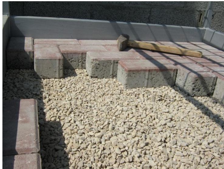
Figure (3.18): Interlock pavement and bedding material
