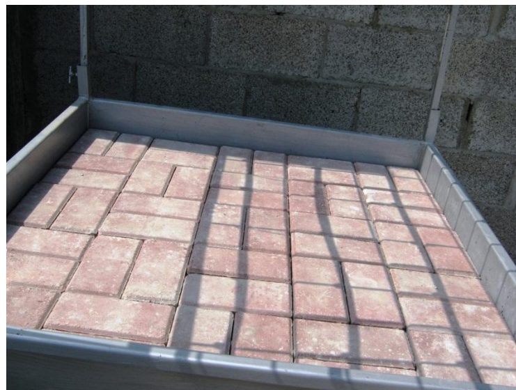
Figure (3.19): Installed pavement surface
